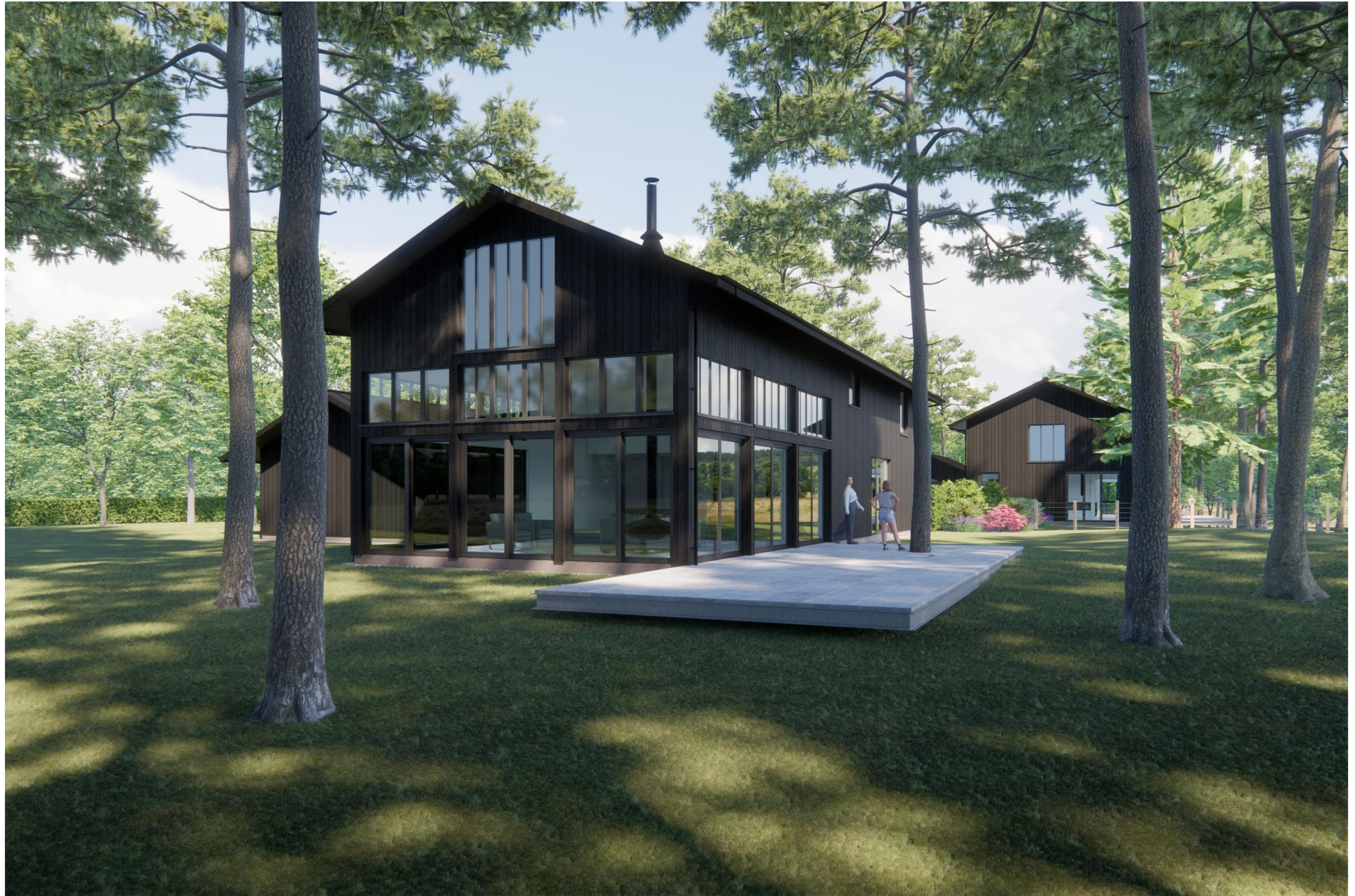
view looking east across house 2 south and west elevation
