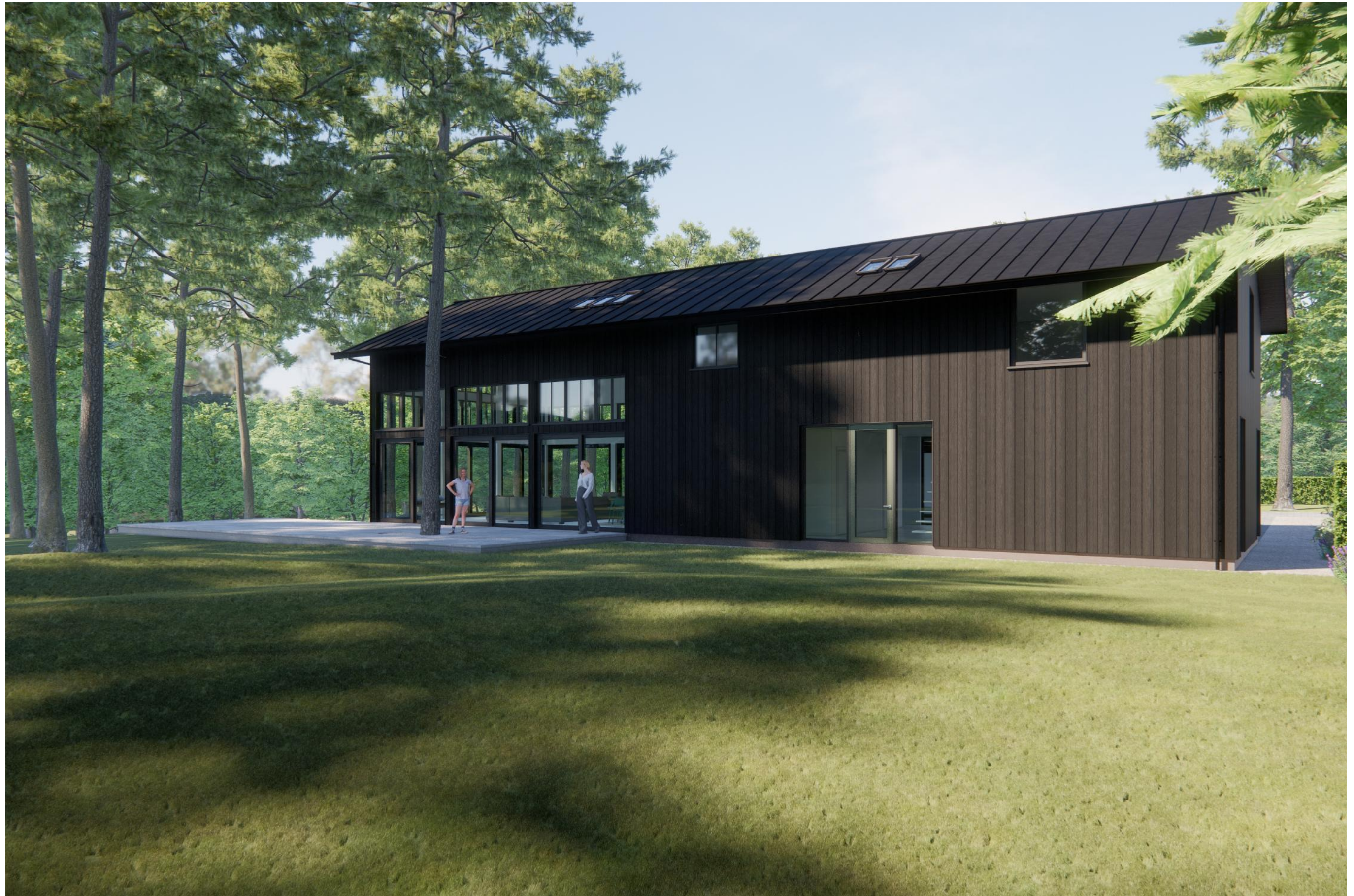
view across house 2 south elevation
