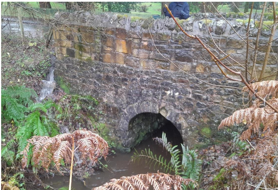
Figure 2: Upstream face of the Knockbuckle Road Bridge over the Gowkhouse Burn
