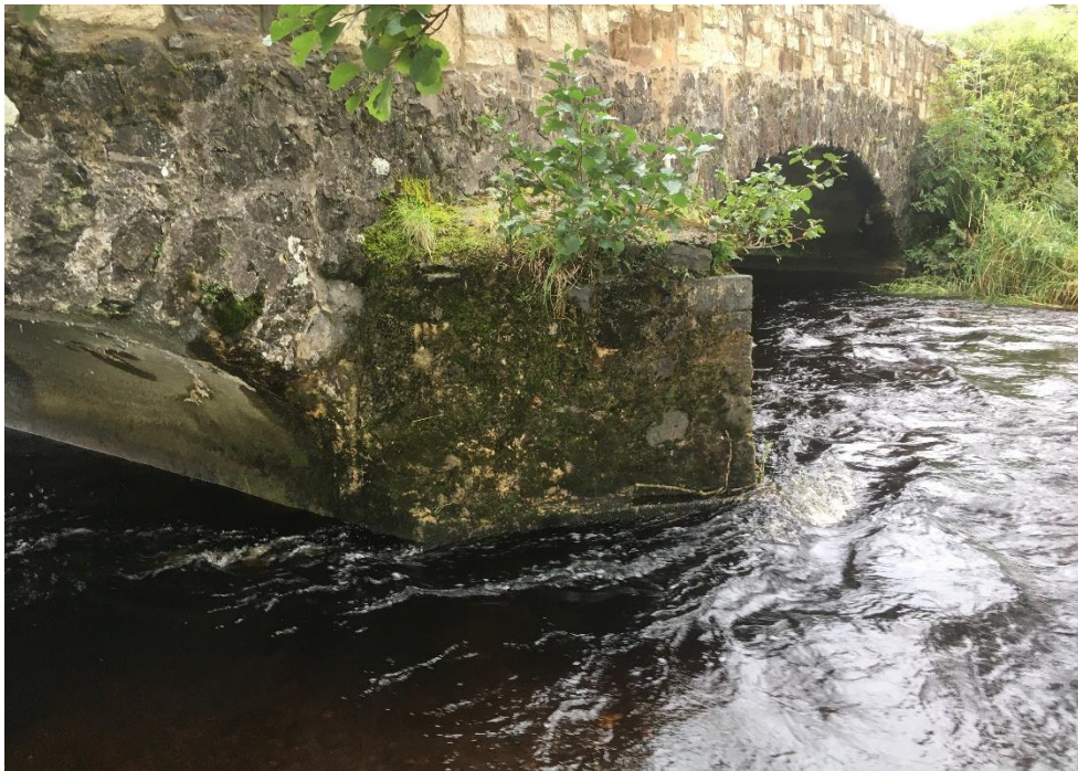
Figure 1: Upstream face of the Netherwood Bridge over the River Gryfe
